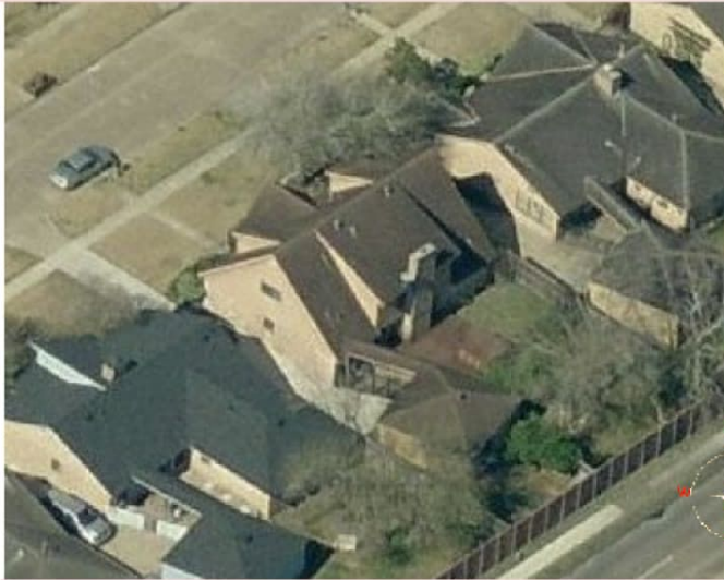
North Side View
