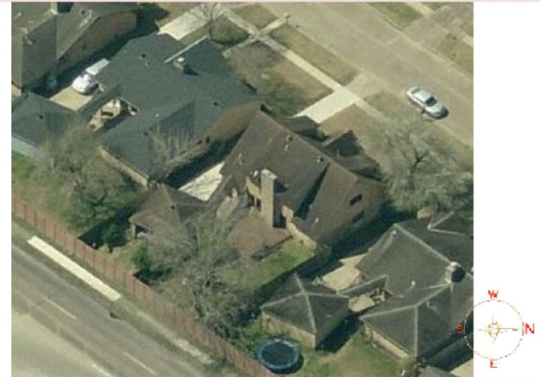
West Side View
