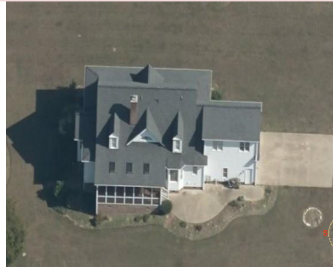
West Side View
