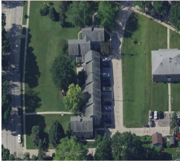
North Side View
