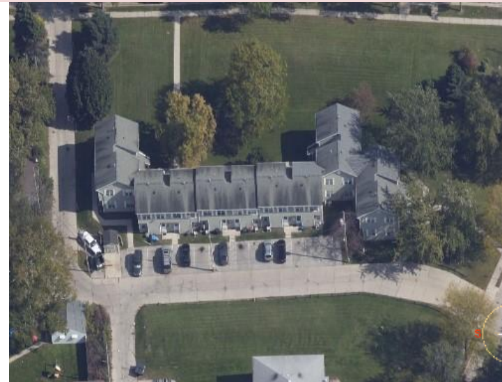
West Side View
